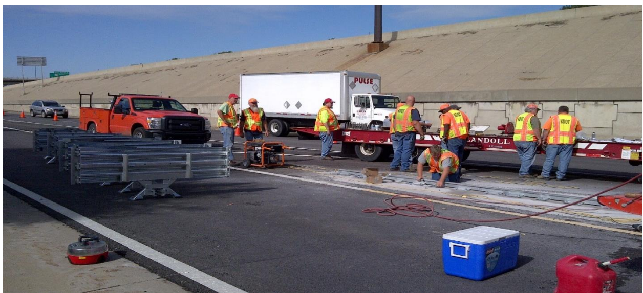
Figure 45. Location 4 Intellicone Portable Site Alarm Deployment near Work Activity
