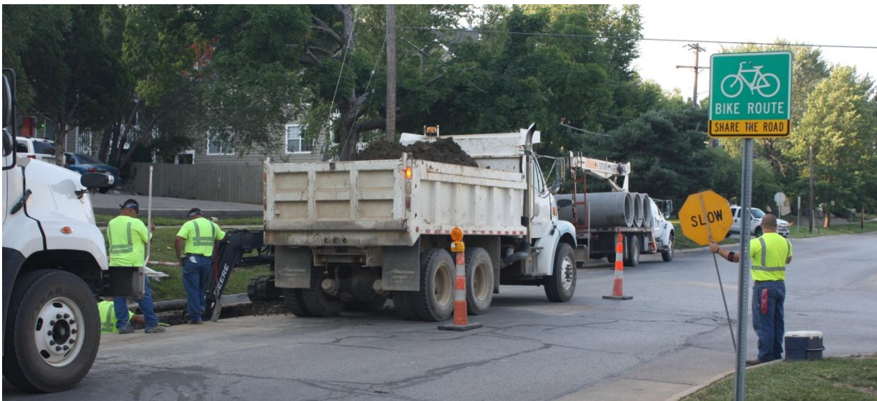
Figure 35. Location 1 Intersection and Work Area with Equipment
