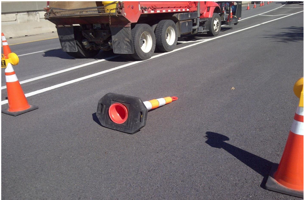
Figure 46. Location 4 Intentional Activation of SonoBlaster Alarm
