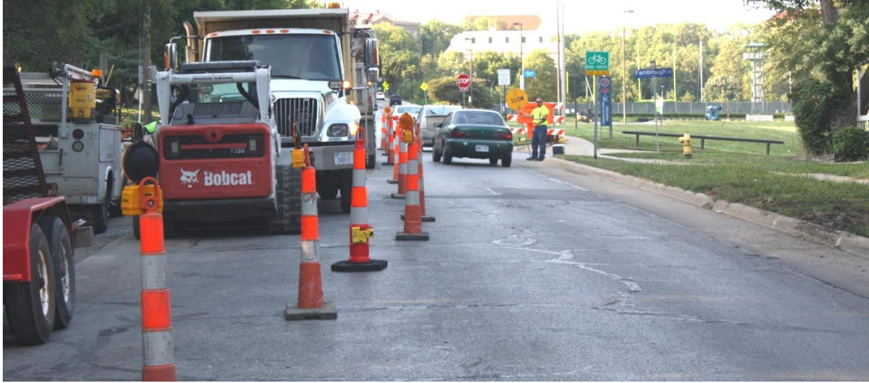
Figure 34. Location 1 Taper with Equipment
