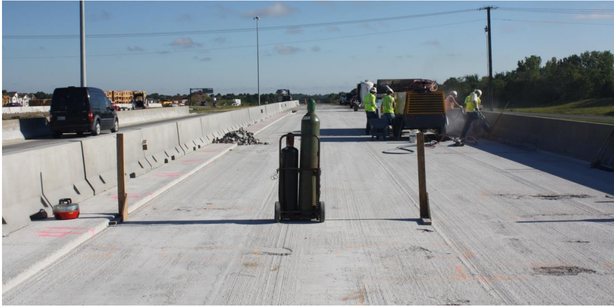
Figure 38. Location 2 Intellicone Portable Site Alarm Deployment near Work Activity
