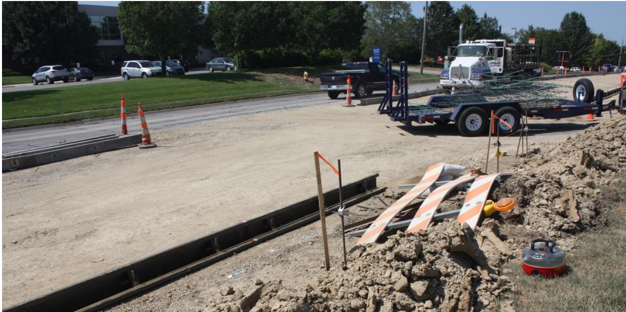
Figure 41. Location 3 Intellicone Portable Site Alarm Deployment near Work Activity
